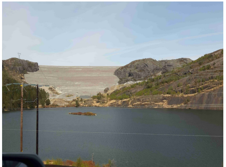
This is Logsvatnet. We see landfill of masses after the ilmenite production of Titania.
