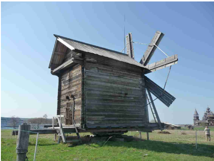
Wind powered grain mill. It stands on a rotatable base, so it is possible to adjust it to the actual wind direction.
