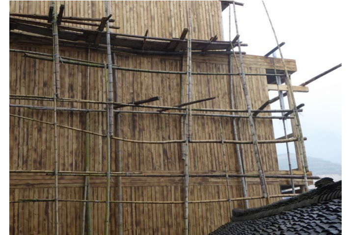
The next day we see how bamboo is used for scaffolding.
