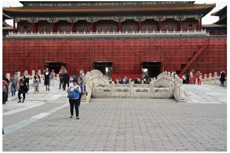
Looking towards The Meridian gate from the inside.
