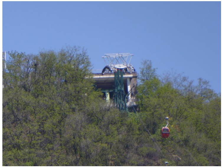
We can also see a bit of the lift.
