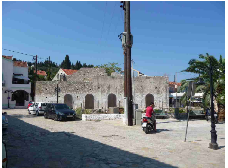
This is probably a ruin from the earthquake in 1953.
