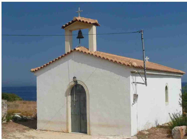
The church, Aghios Giorgios. It was rebuilt after the earthquake with some of the stone from the temple.
