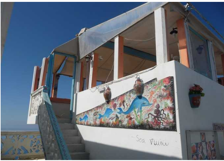
When we came up here, it turned out that the restaurant was closed for the winter, and they had started renovations.
