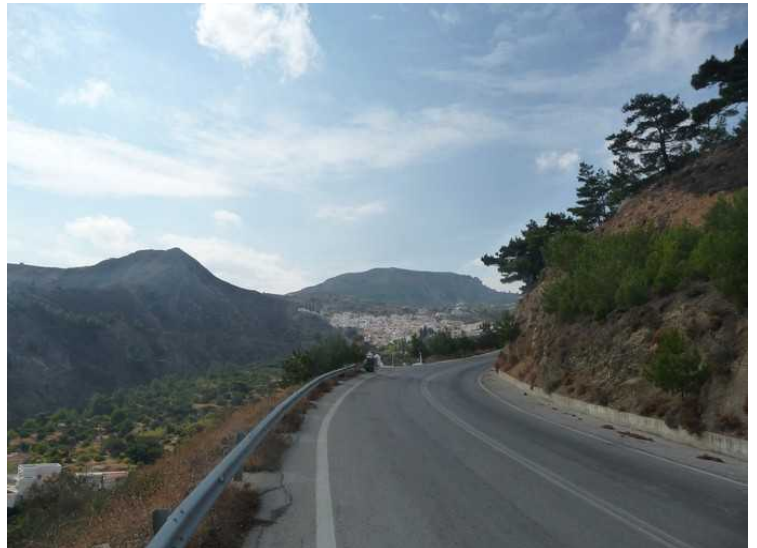
The road is in the hillside above the town.
