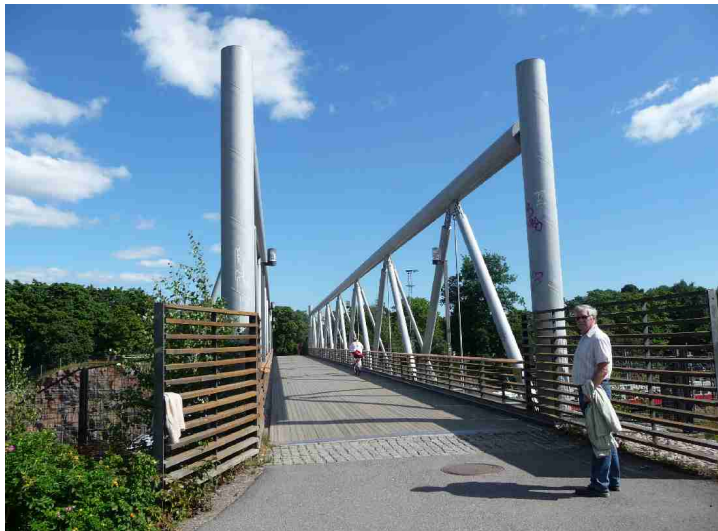
Footbridge over the railway.
