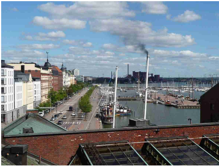
A view towards the north part of the harbor.
