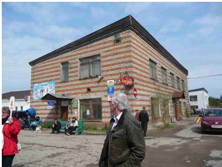
The bus station in Kirillov.
