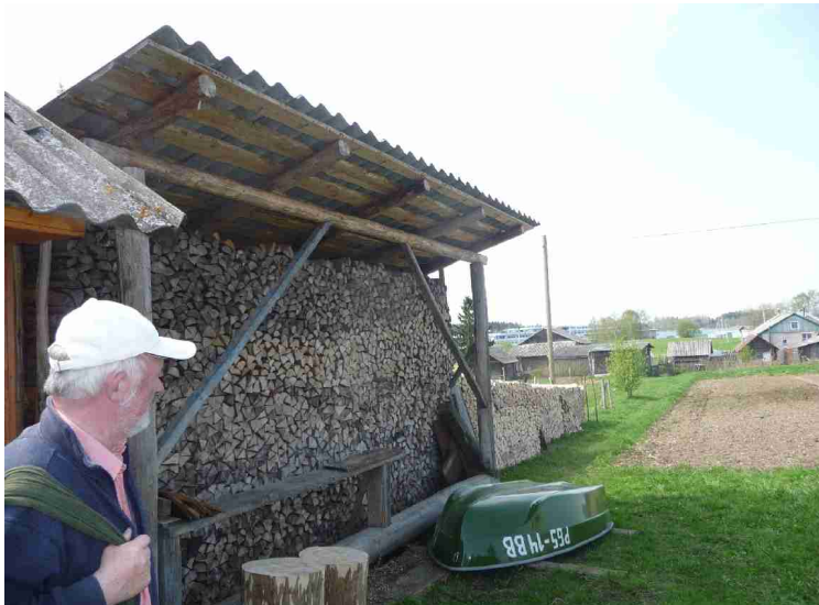
The wood store is calculated to last for 3 years. They have also installed electricity.
