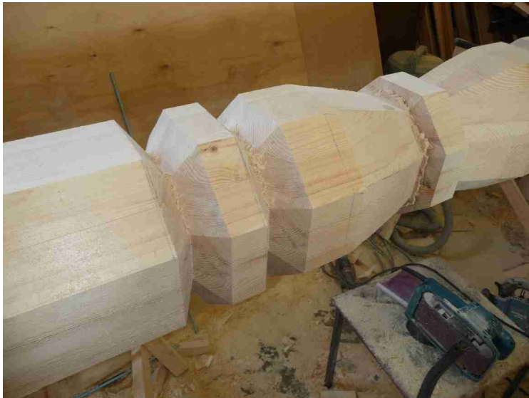
The have started the processing of a column.
