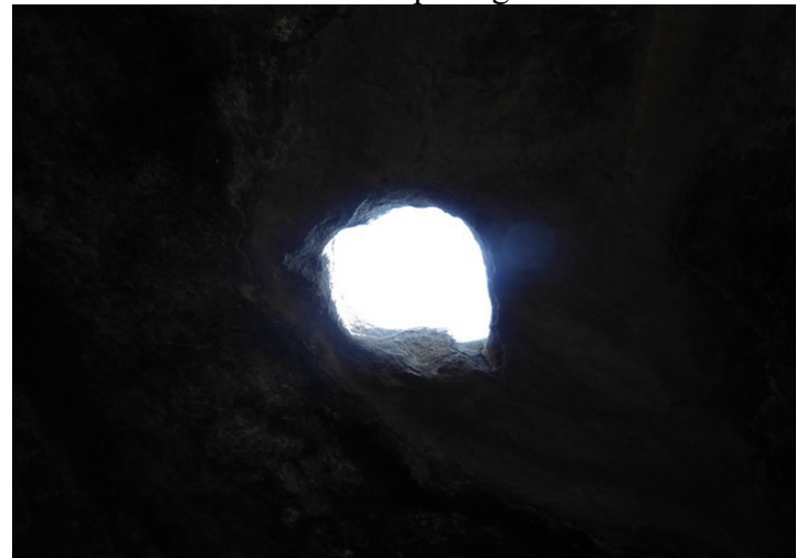
The rain comes in through this hole in the roof.
