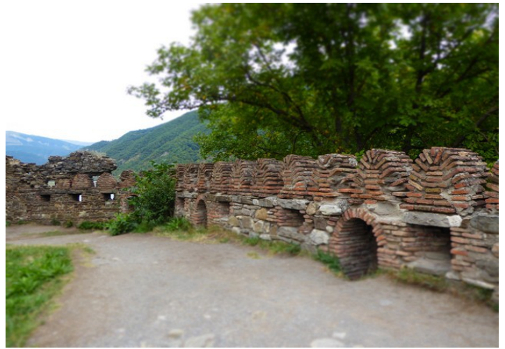
The walls from the inside.
