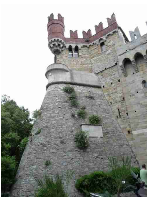
Some of the walls seen from outside
