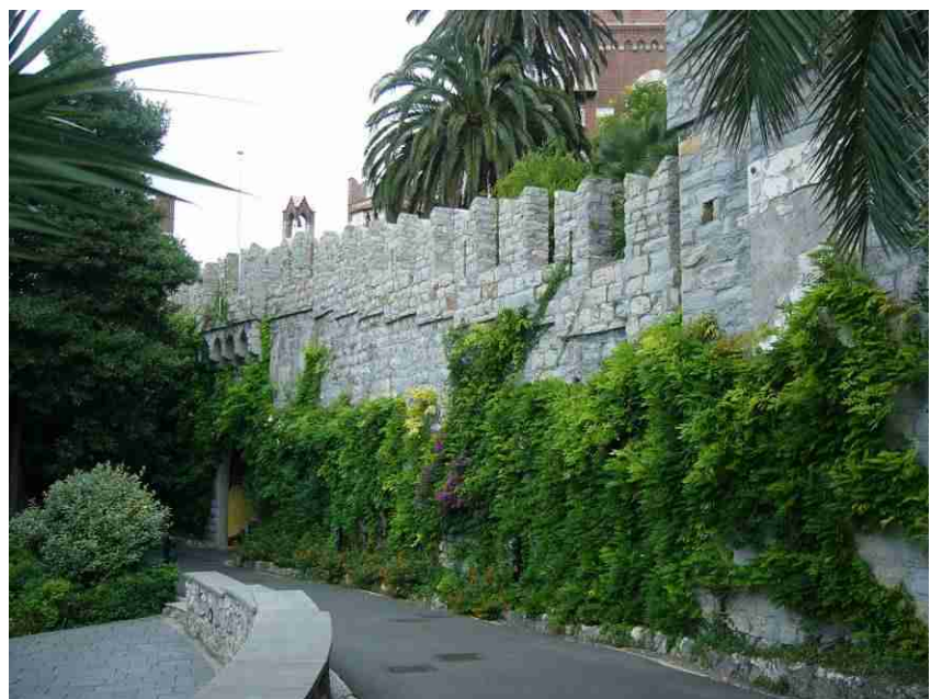
There is also walls inside the walls
