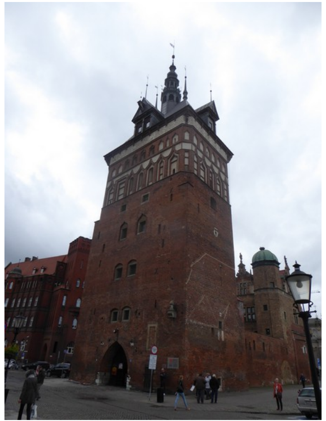
We left the driver at Targ Węglowy. Here is the Amber Museum . Before that there was a prison tower and torture chamber.
