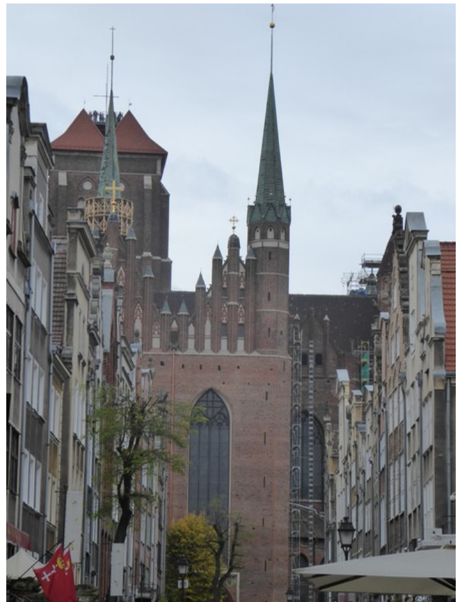
In the end of the street lies St. Mary's Church
