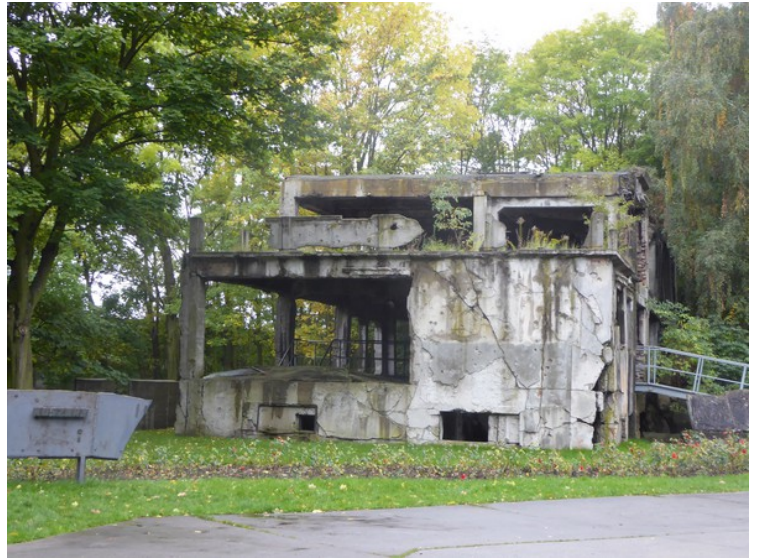
One of the barracks is part of the museum.
