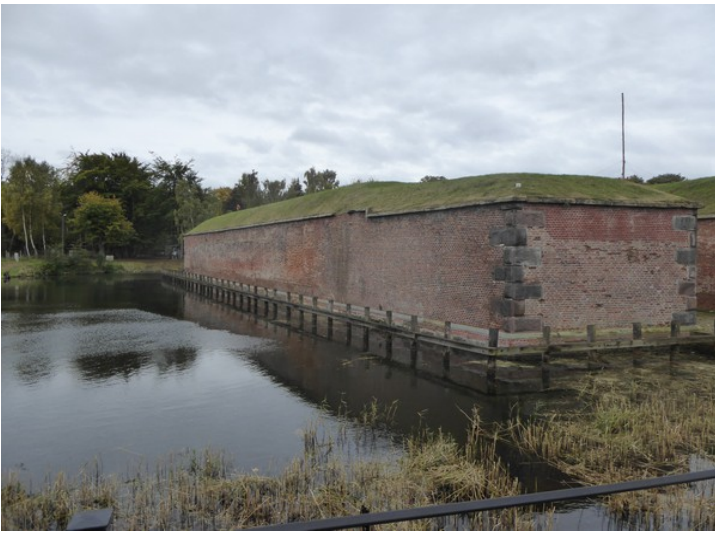
The moat on the other side of the entrance.
