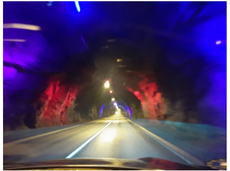
Norðoyatunnilin was opened in 2006. It links Leirvík on Eysturoy with Klaksvík on Borðoy . It is 6300 m long. In the middle of the tunnel there is so-called light art.
