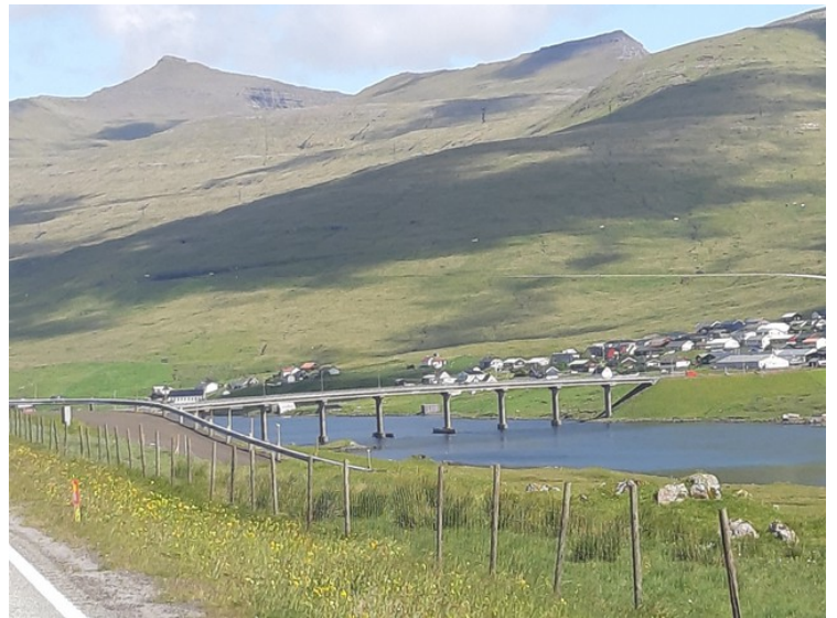
Here we see Streymin Bridge . It joins Streymoy and Eysturoy and was completed in 1963.
