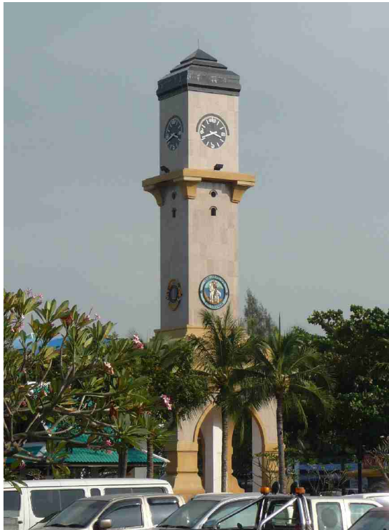
A nice staple tower.
