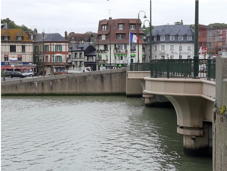
This is the bridge that crosses the river between the two districts.
