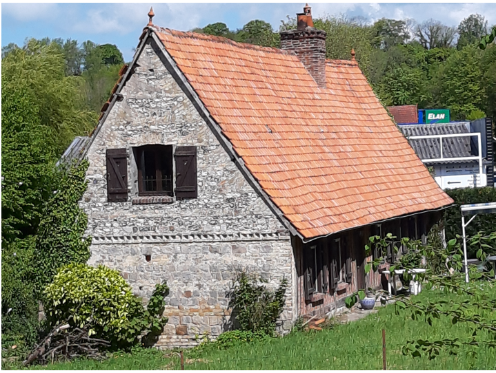
Nice house by the road.
