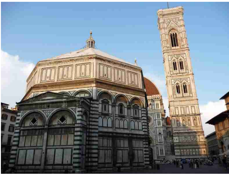
The baptistry, Battistero di San Giovanni, and Florentin Giotto's clock tower (85m high) stand in front of the cathedral.
