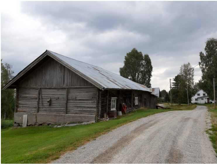
Operational building and residential house on Rotberget.
