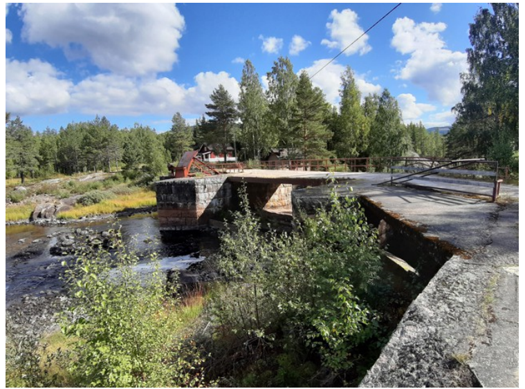
The dam seen from upstream.
