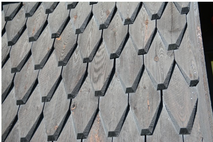
Walls, towers and ceiling are covered with ca. 50,000 profiled shavings.
