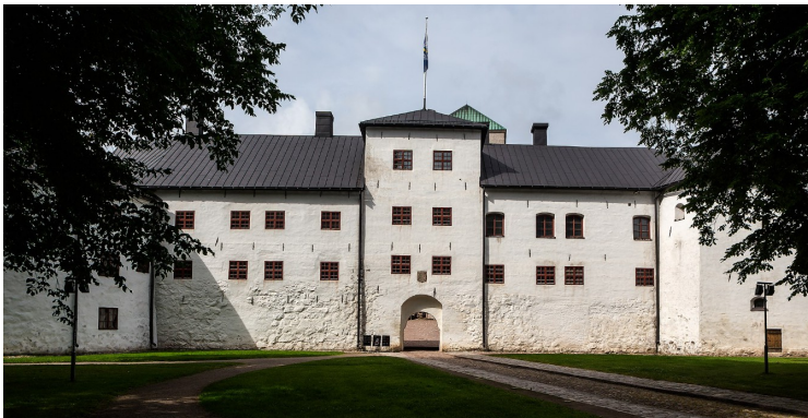
This is the eastern facade.
