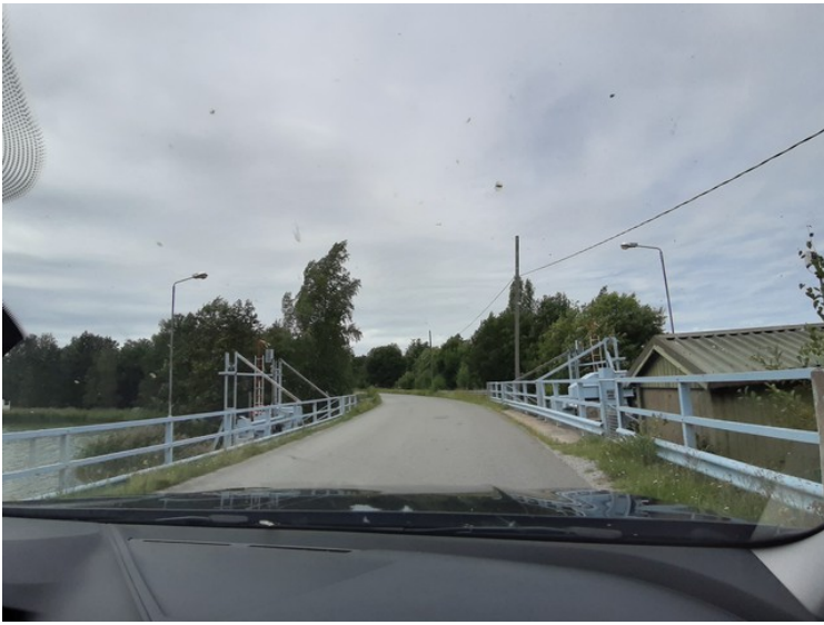
This is Simonbyslussen. The lock was built in the 1960s. It separates seawater and fresh water inside the fjord on the island. Small boats can go through the lock. It is inspected in spring, summer and autumn.
