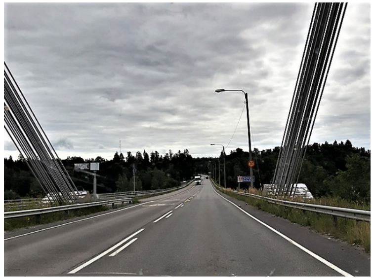
Here we drive on the Rävsundsbron from Kustö over to Kirjala . The bridge is the longest suspension bridge in Finland.
