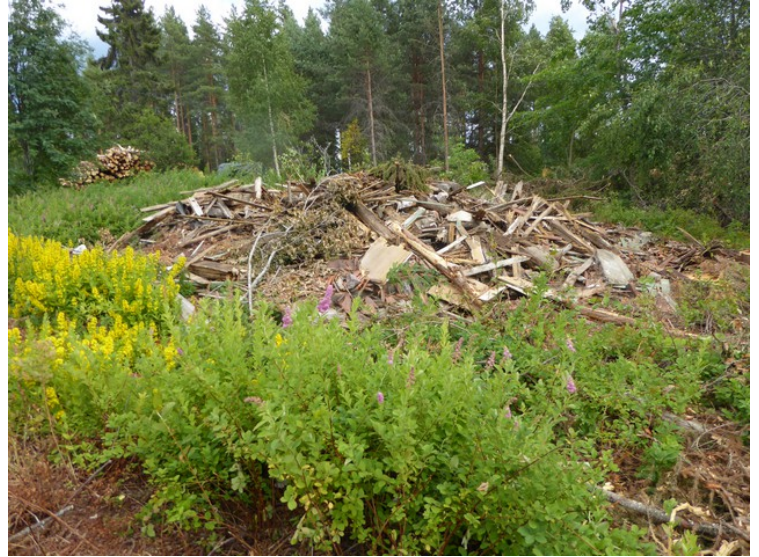
It was torn down during the winter, so now it's just this pile left of the house.
