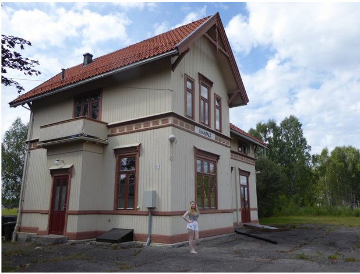
The station building at Namnå. It is only freight trains that run here now. Passenger services were ended in 1994.
