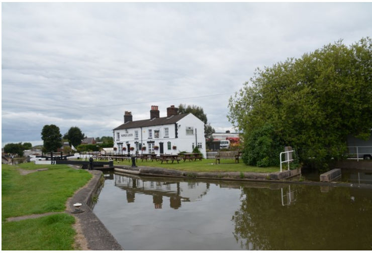
The last thing that has happened in the lock, is that a boat has gone up. Then the lock chamber is full of water, and it is ready for the boat to go right in.
