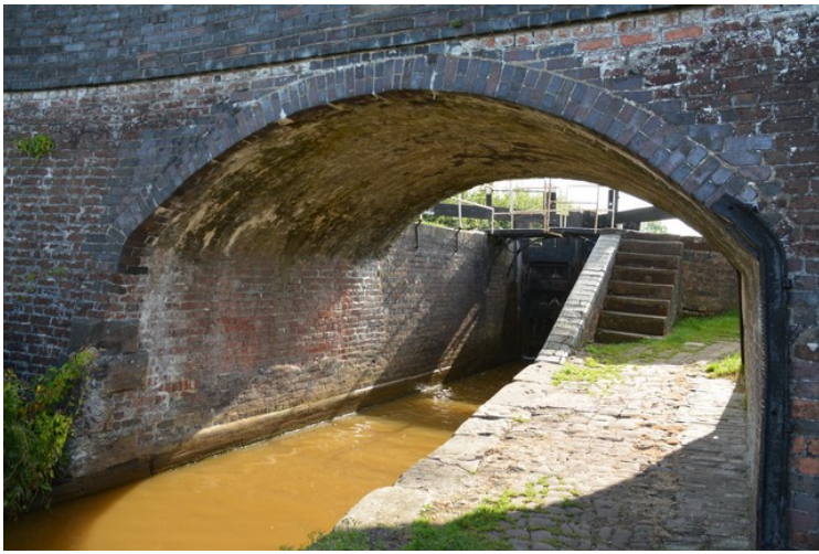
A lock with shut gates.
