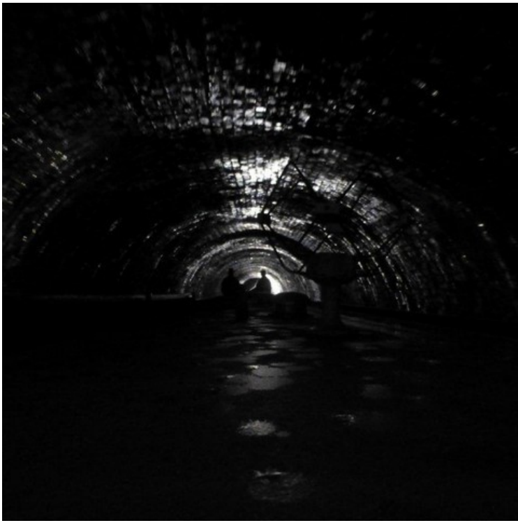
We have a boat behind us and it lights up the ceiling of the tunnel, so when we look from bow to back, it looks like this.
