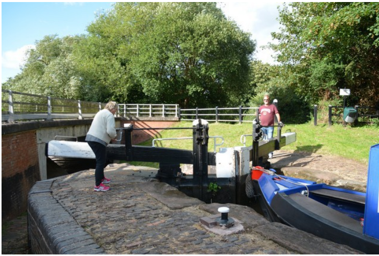
Here Anni and Eldor is opening the lock paddles on either side to let the water out of the lock chamber.
