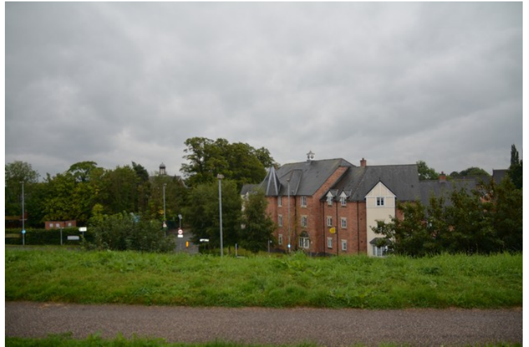
Here the canal is built above the adjoining land.
