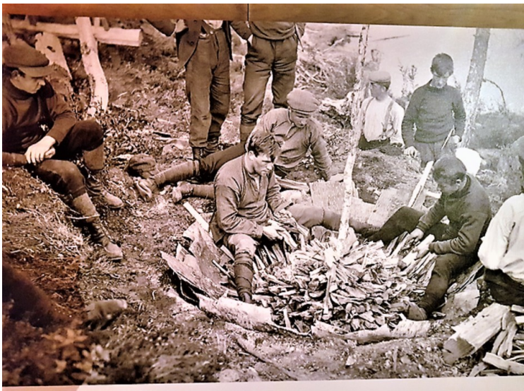
Preparation for tar burning.
