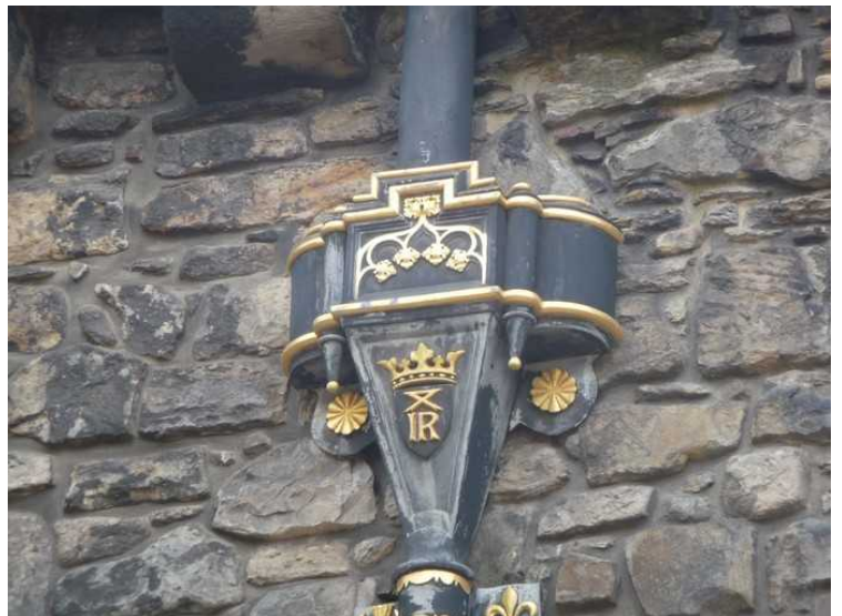
The top of the pipe.
