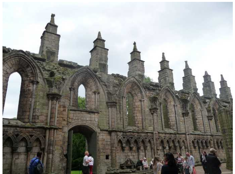
The walls are still impressive.
