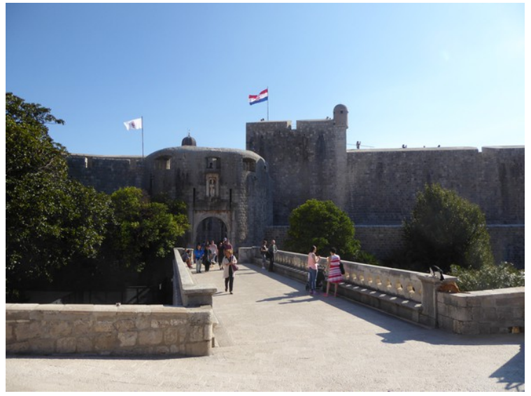
This is the bridge crossing the moat to the main gate, Pile . There are 4 gates in the city wall. This is most used.
