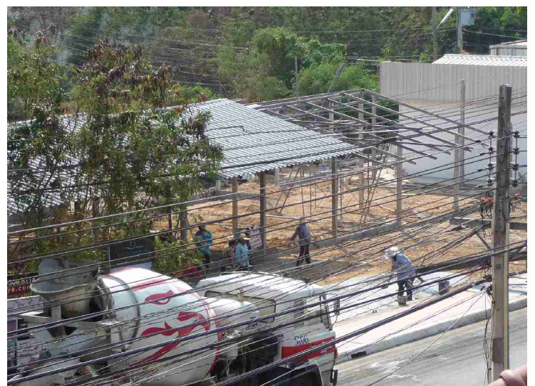
The ready-mixed concrete is coming. The concrete is put directly on the ground.
