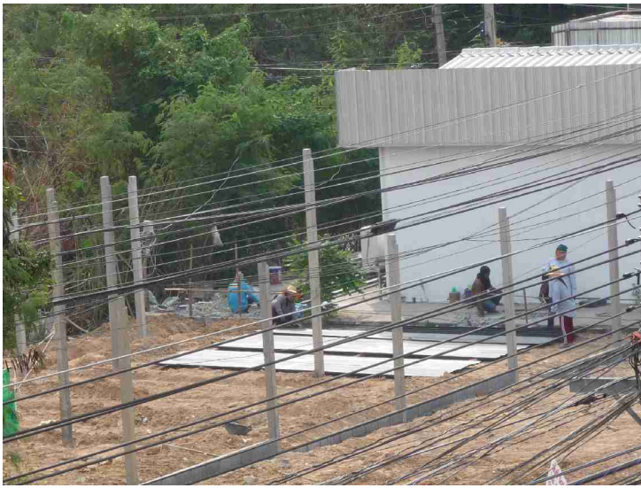
Roofing sheets have started to arrive.
