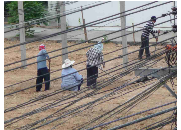
Then the ground is leveled.
