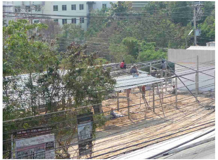
Here the mounting is well under way.
