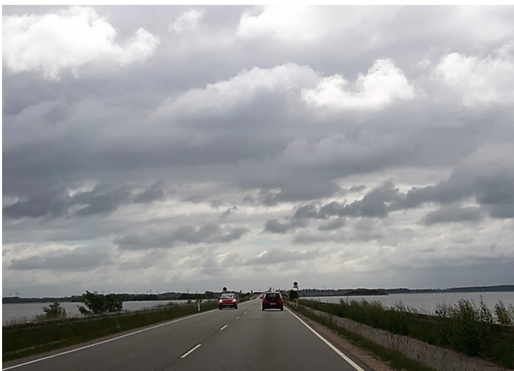
The road further towards Langeland goes on embankments in the sound and on a low bridge.
