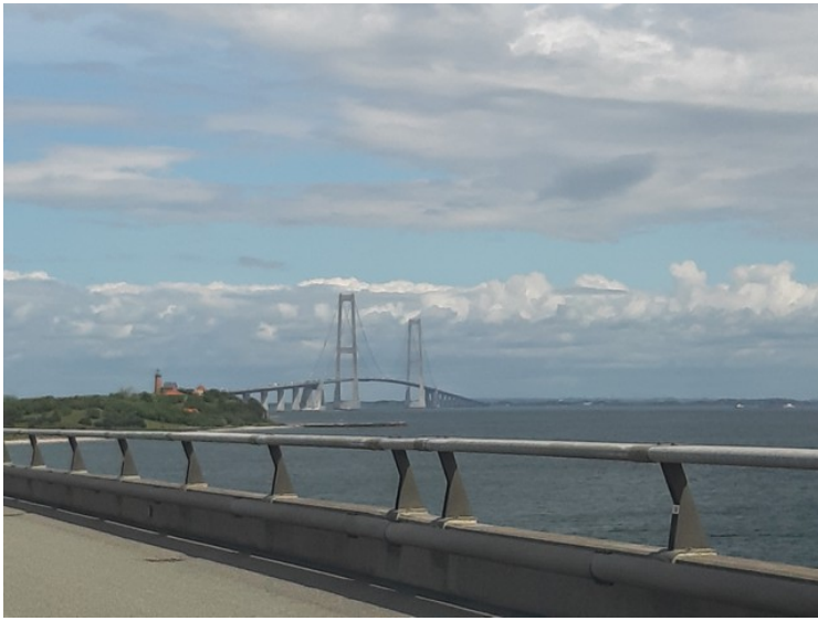
Here we drive across the Great Belt. We are on the West Bridge and looking towards the East Bridge. The Great Belt Fixed Link connection was opened in 1998.
