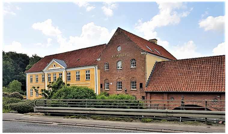
This is the Rye Mill . It was built in the 16th century. There has been a grain mill and later a wood grinding mill and most recently a clothing factory. From 1971, the mill has been used for electricity production. This is still going on.
