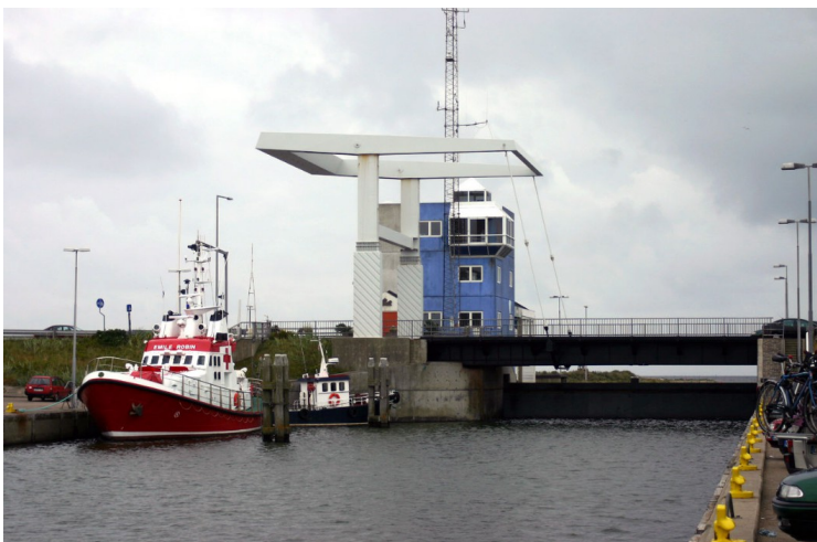
This is the second part of the lock system. It is a chamber lock with an associated tilting bridge. It allows passage between the North Sea and Ringkøbing Fjord.
