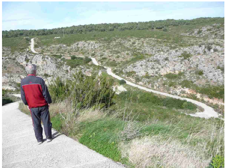
There is concrete covering in the steepest hills.
