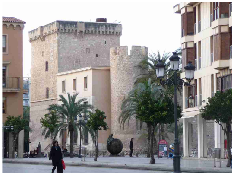
Here we see the fort from the church square
