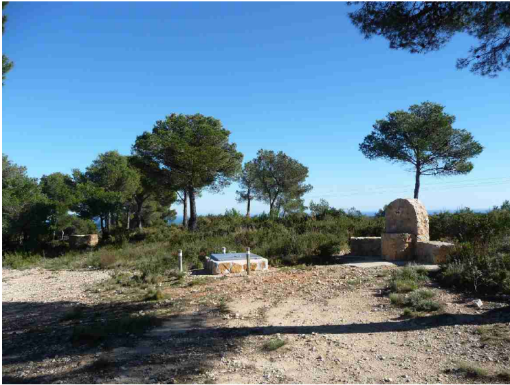
There were water posts and connections for fire hoses along the path.
