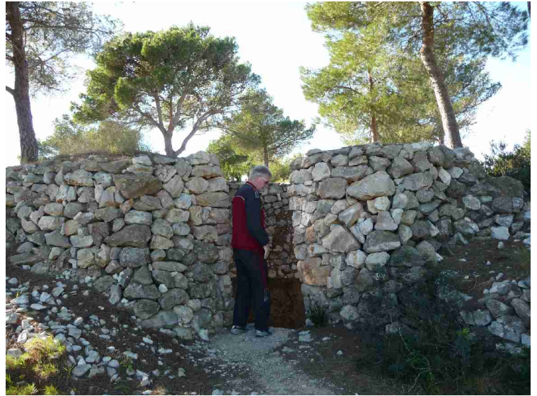
Kjell is not peeing. He is looking down into a big water reservoir.
