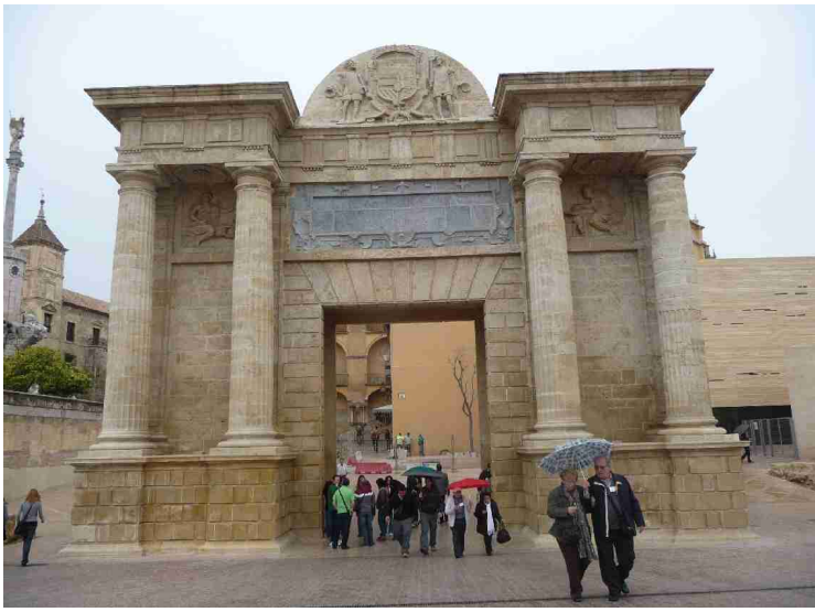
This is Puerta del Puente seen from the bridge.
