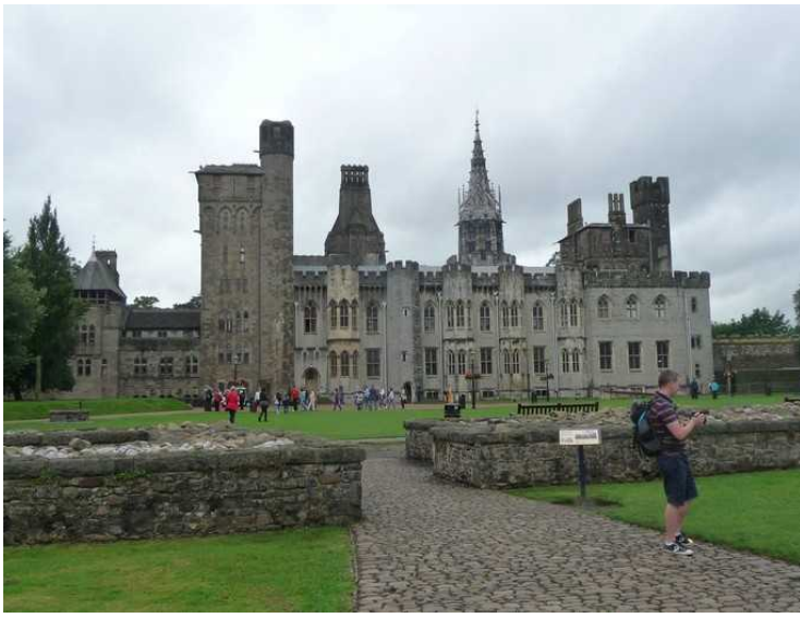
The palace is also located within the walls of Cardiff Castle. It was built in the years 1423 - 1439, but has been altered and extended many times after that.
