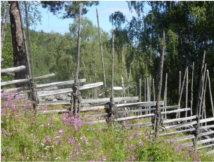
The roundpole fence is mounted with withe twigs.
