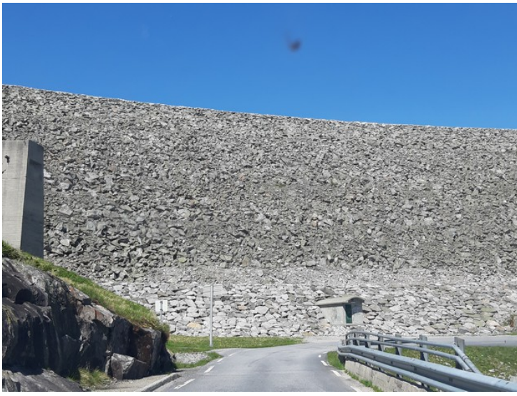
This is the dam in Rosskreppfjorden .
