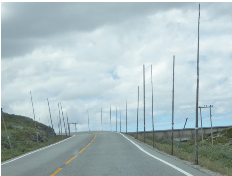
After Haugastøl, the road crosses Hardangervidda . Here the piers are tight. It looks like they're up all year.
