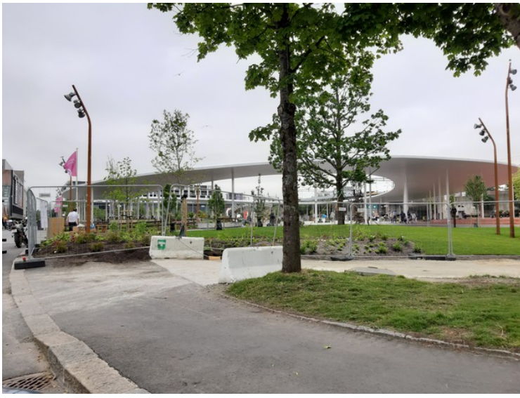
The bus station in Sandnes has been upgraded this year. What shows best is this circular roof.
