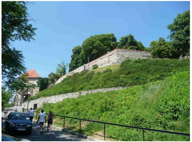
View upwards, towards the gate.
