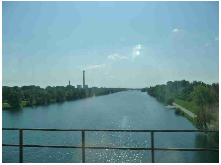
New Danube is a side arm of Danube that is used for regulation of the water level at high water.
