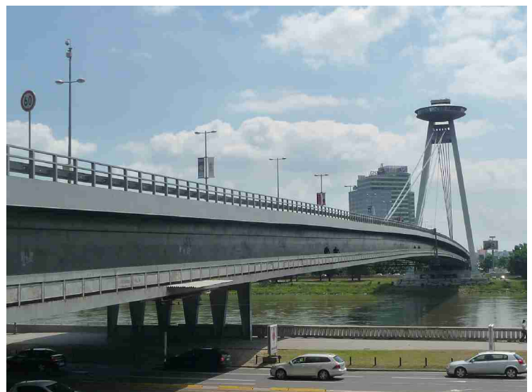
Nový Most (New bridge). In the top of the pylon, which is 84.6m tall. There is a ufo like restaurant.
