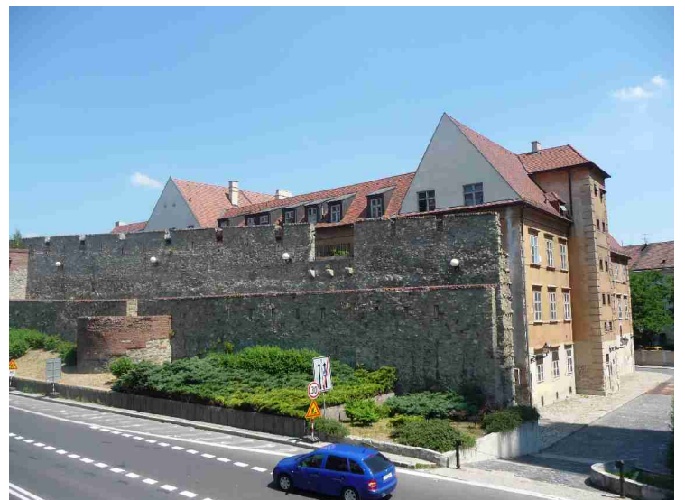
Remnants of the town walls.
