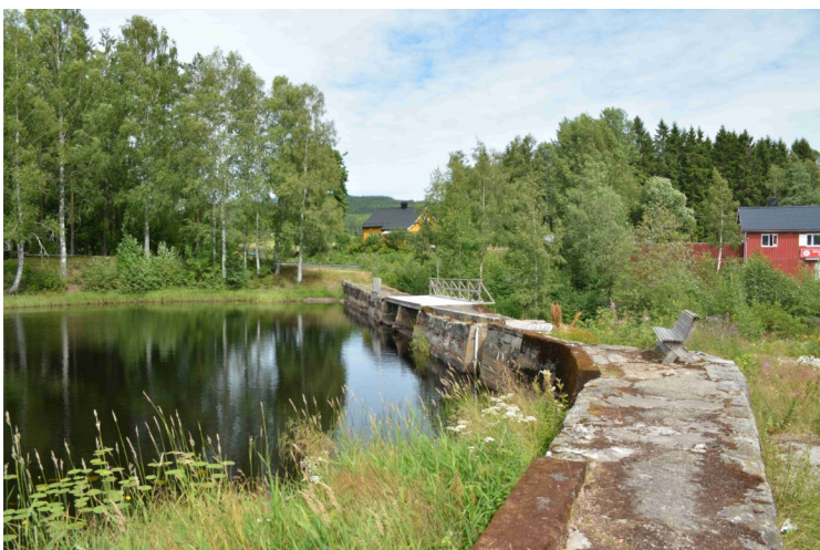
This is the dam. It is about 100 m long with two dam hatches, two floodgates, a bottom hatch and a float channel. It has been well maintained.
