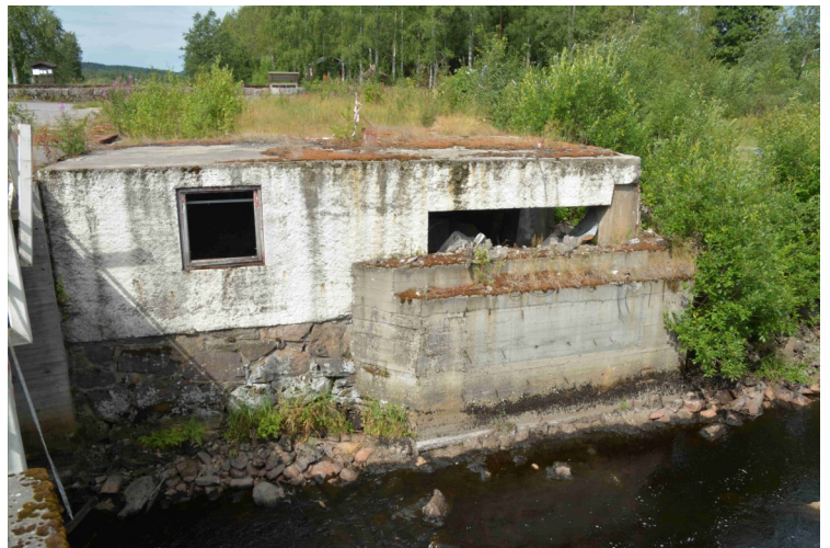
This foundation remains.
