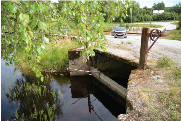
One of the dam hatches.
