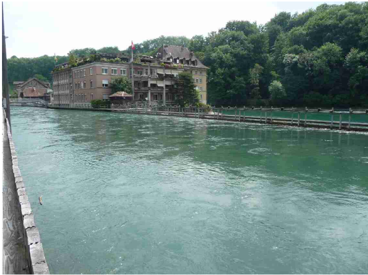
We can see the dam on the far side.
