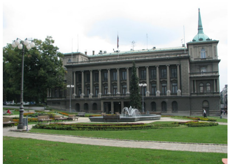
Right next to the old castle lies The New Castle . It was built in 1911-22. It was used by King Alexander. Today it is used by the president of Serbia.
