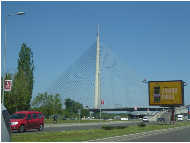
This is the bridge pylon of the newest bridge over Sava, Ada Bridge . The height is 200m.
