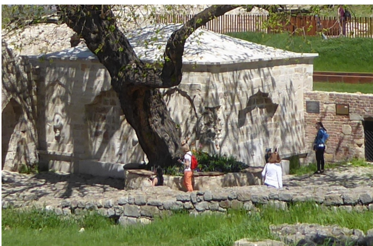
This is Mehmed Paša Sokolovićs Fountain , a drinking water fountain. It was erected in 1576-77. It was buried at one point or another and was not discovered again until 1938.
