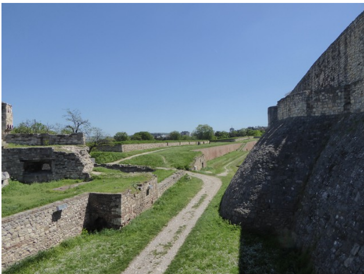
Area between the walls.
