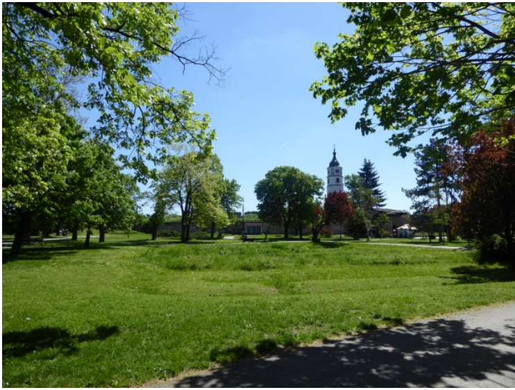
The clock tower seen from a distance.
