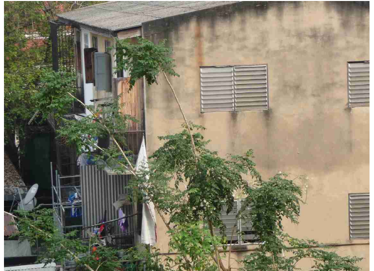
There is obviously not much spare money for maintenance.
