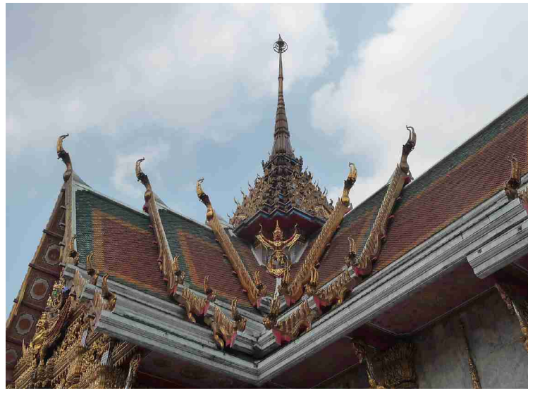
Details from a roof.
