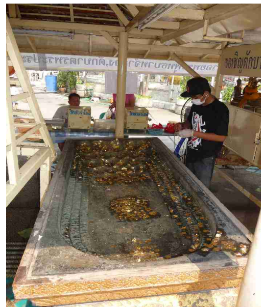
This is a decoration, which is repaired. There is lacking some leaf gold here and there.
