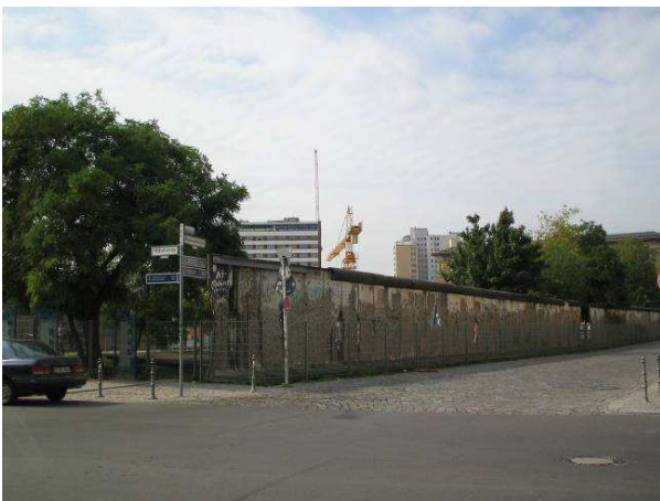
Right beyond, there was a whole section of the wall that was preserved.
