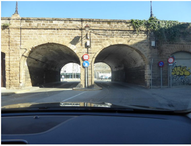
Here we are driving through the wall.
