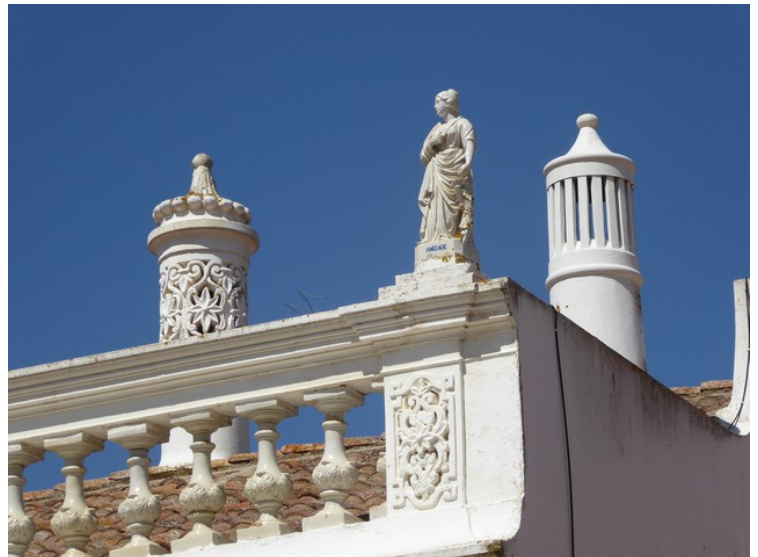
The entire Algarve coast is known for having nicely decorated ventilation pipes.
