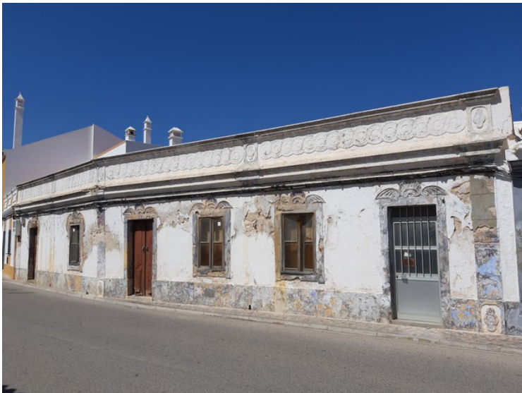
This building has been nice once.
