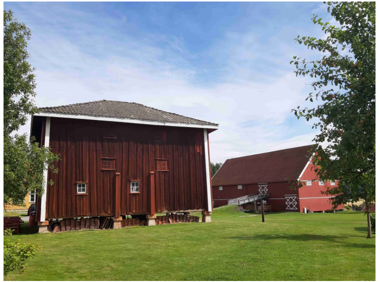
The store house has three floors. It was used as a granary in the 18th century.
