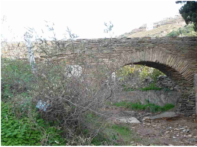
A nice footbridge across the brooke. It is dry just here.
